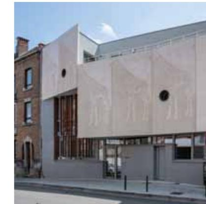
wants even more individuality. As you would expect, NOE Schaltechnik is delighted to receive these requests and works closely with the customer to come up with some sensational NOEplast motifs. They are always completely in accord with the design requirements for each specific project.
