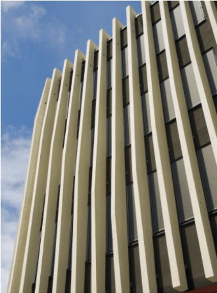
The surface of the lisenen looks like the natural stone travertine. This appearance was created by placing NOEplast textured formliners in the precast concrete unit forms. Architect Zurmöhle remarked: "... the concrete surface always looked simply perfect."
