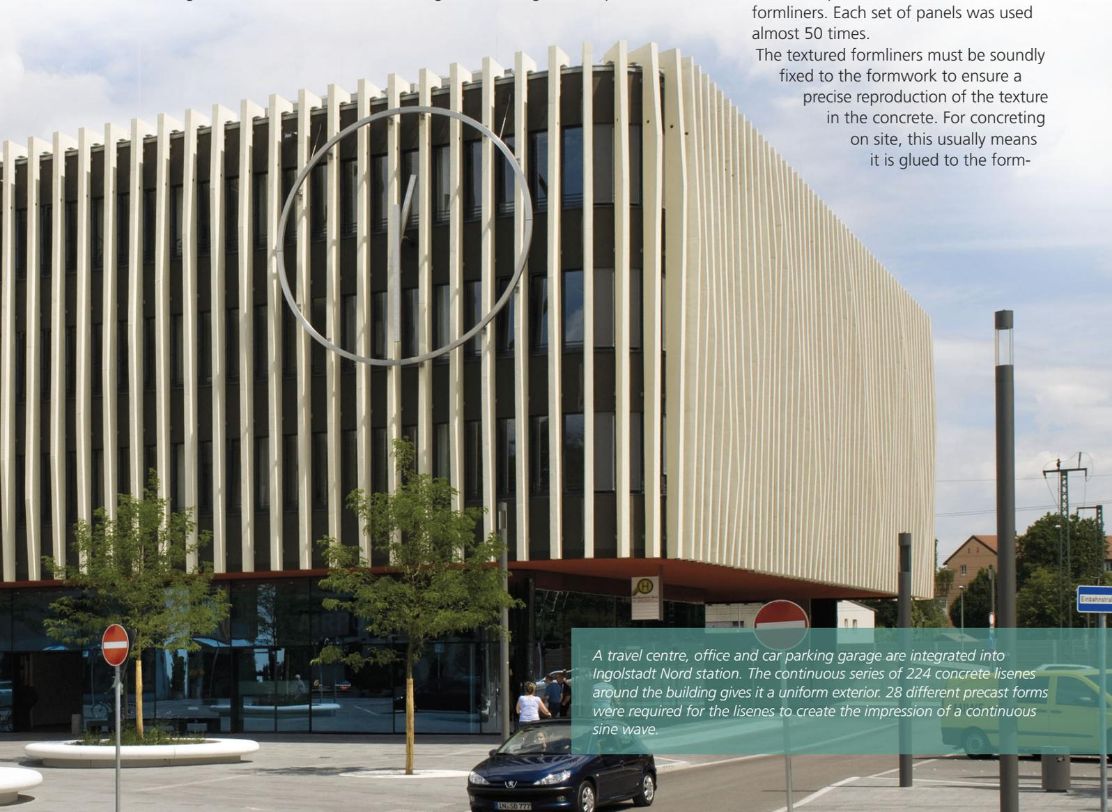
*A travel centre, office and car parking garage are integrated into Ingolstadt Nord station. The continuous series of 224 concrete lisenen around the building gives it a uniform exterior. 28 different precast forms were required for the lisenen to create the impression of a continuous sine wave.*
