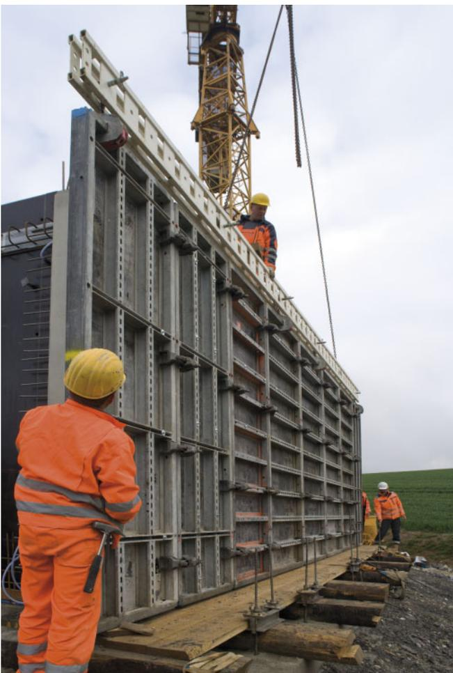
*A NOEtec girder made it easy for the site team to erect and strip the formwork.*
