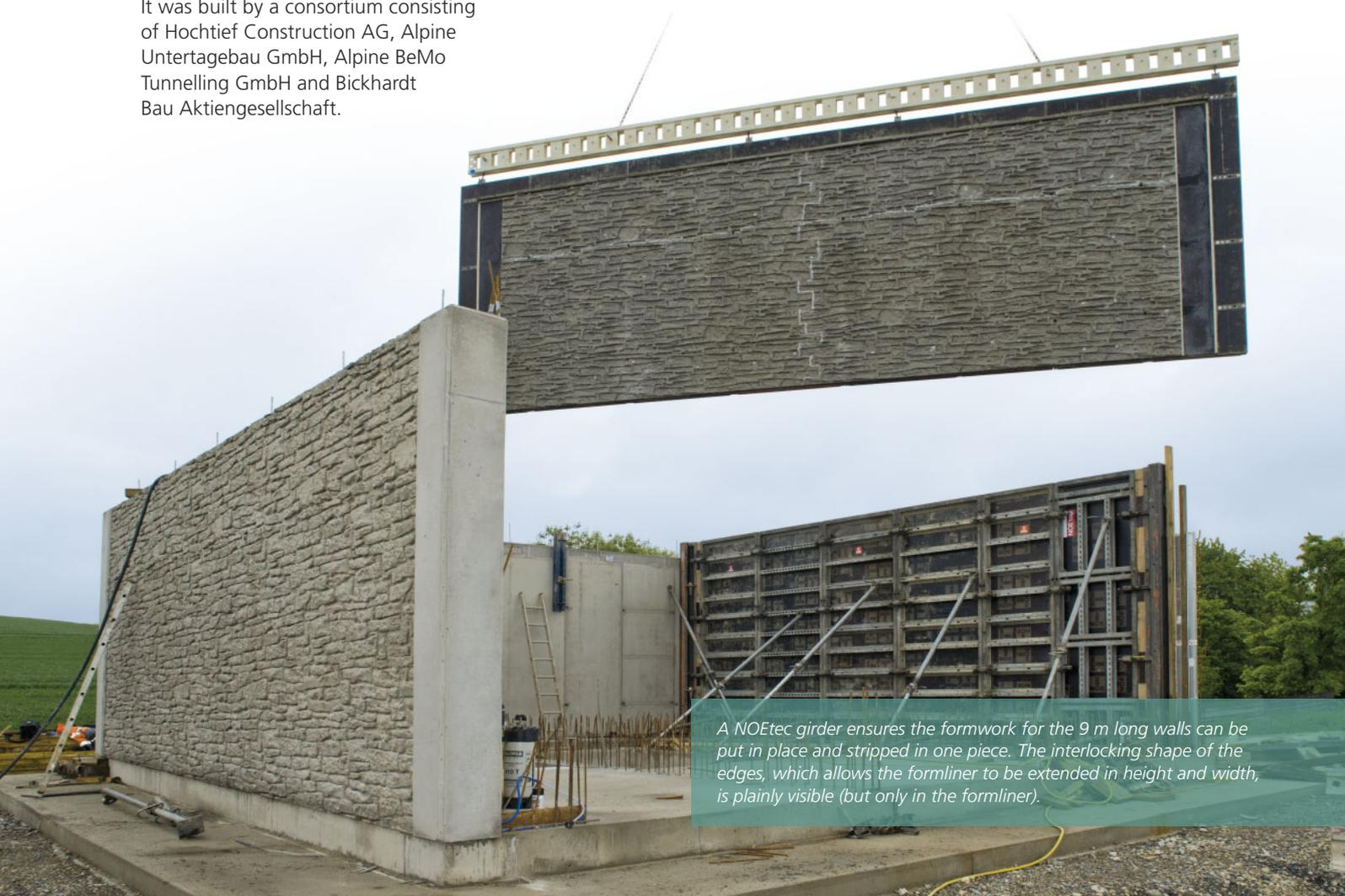
*A NOEtec girder ensures the formwork for the 9 m long walls can be put in place and stripped in one piece. The interlocking shape of the edges, which allows the formliner to be extended in height and width, is plainly visible (but only in the formliner).*
