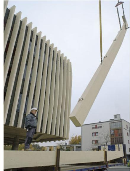
A logistical challenge: the transport and installation of the 13 m plus long lisenen on Ingolstadt Nord station in possibly windy conditions.
