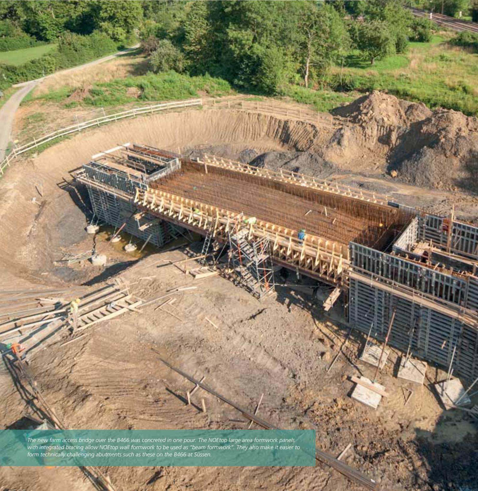
*The new farm access bridge over the B466 was concreted in one pour. The NOEtop large area formwork panels with integrated bracing allow NOEtop wall formwork to be used as "beam formwork". They also make it easier to form technically challenging abutments such as these on the B466 at Süssen.*
