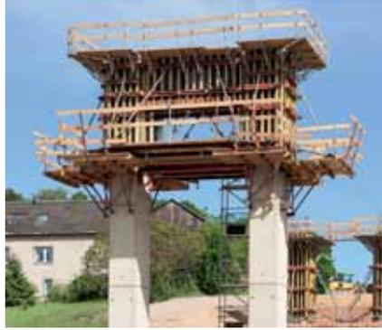
*All the advantages of the NOEratio beam formwork came into play when erecting the forms for the column pair head.*
