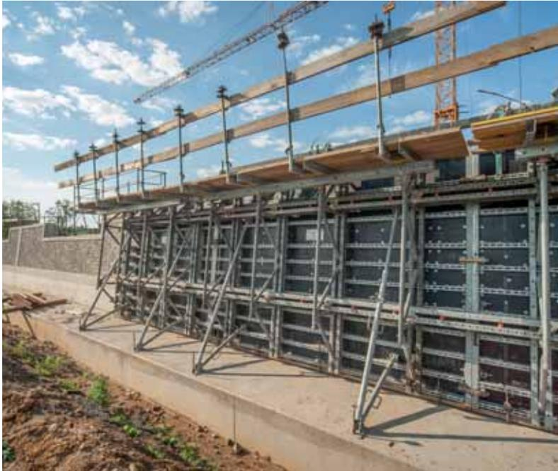
*The panels had a max. size of 300 x 512.5 cm, so that 9.60 m long wall segments could be concreted using only 4 formwork panels.*
