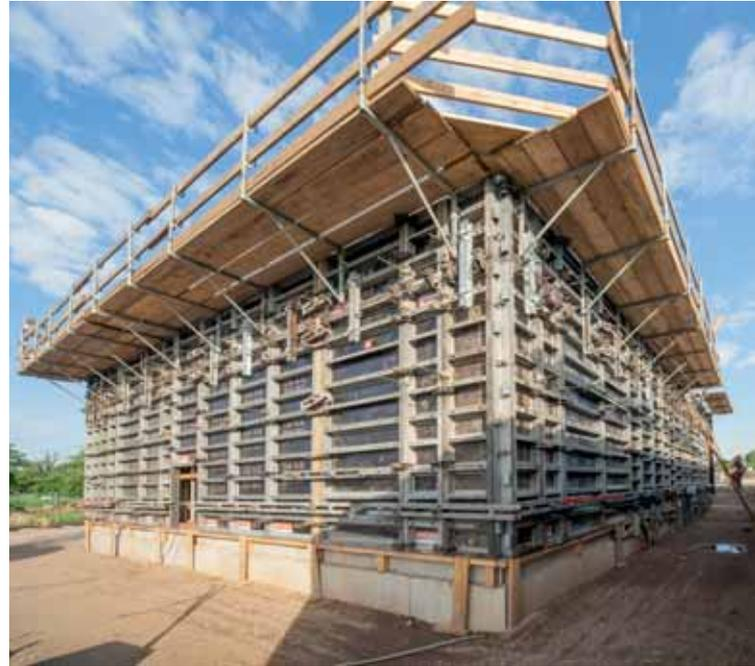
*The contractor decided to use the proven NOEtop formwork system for the pump houses at each end of the Elbe dyke.*
