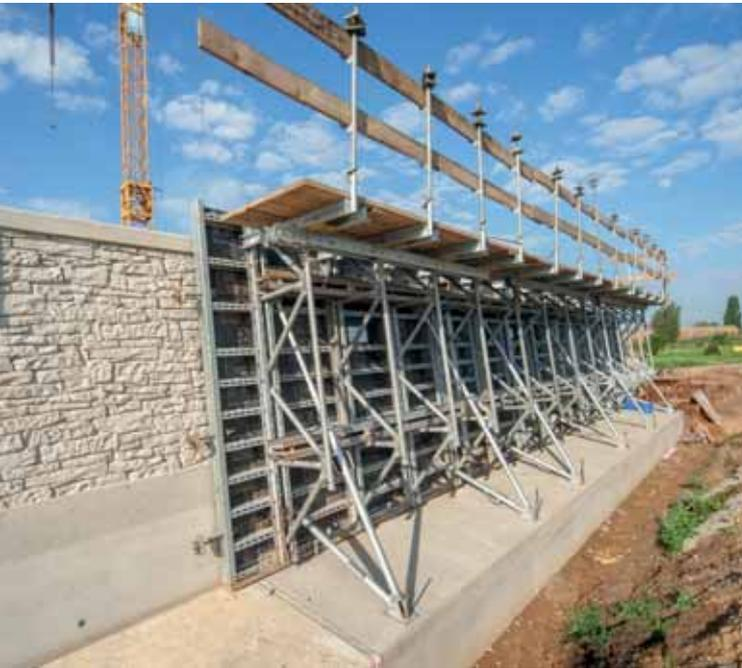
*With the NOE Combi 70 system, the ties were placed in the plinth area and above the formwork. There were no ugly tie bar marks in the fair-faced concrete surfaces.*
