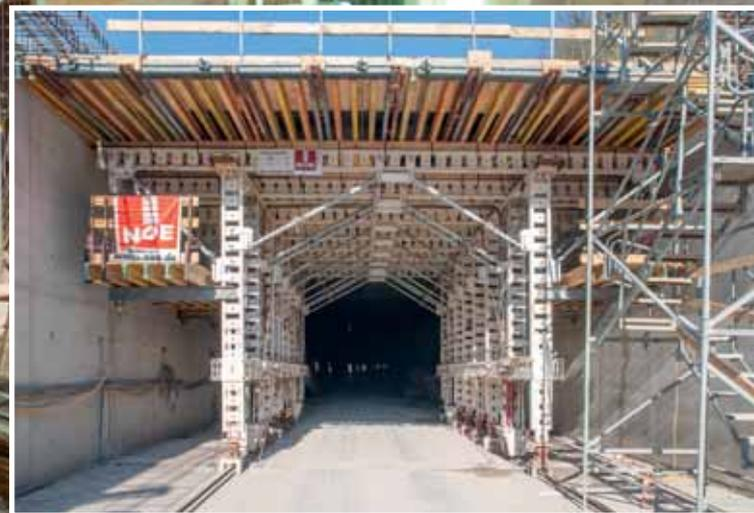
*For concreting the tunnel portal decks, main contractor Ed. Züblin AG opted for a NOEtec Deck formwork carriage.*
