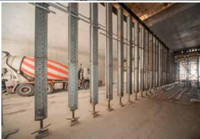
The temporary propping was performed by NOE LS 200 heavy-duty props.
