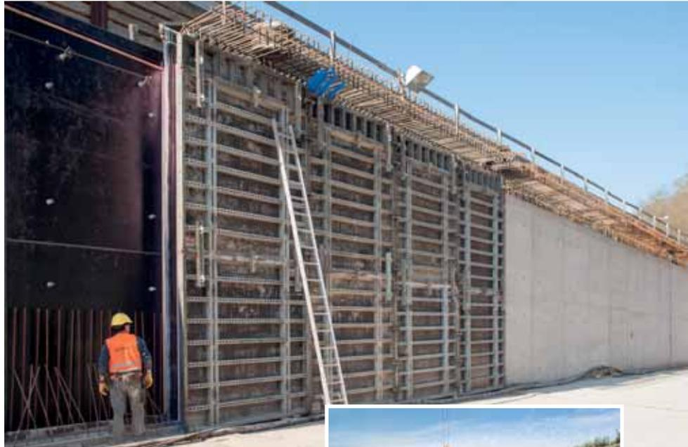
*The tunnel portal walls were poured using NOEtop large panel formwork. The tie bar hole positions can be placed anywhere in the bracing.*
