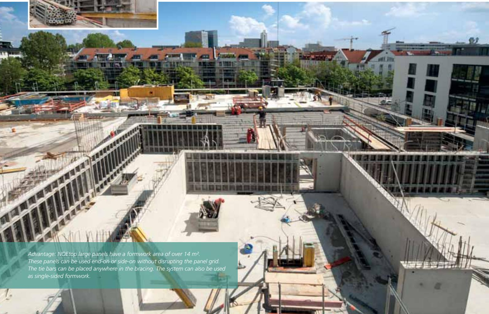
*Advantage: NOEtop large panels have a formwork area of over 14 m<sup>2</sup>. These panels can be used end-on or side-on without disrupting the panel grid. The tie bars can be placed anywhere in the bracing. The system can also be used as single-sided formwork.*
