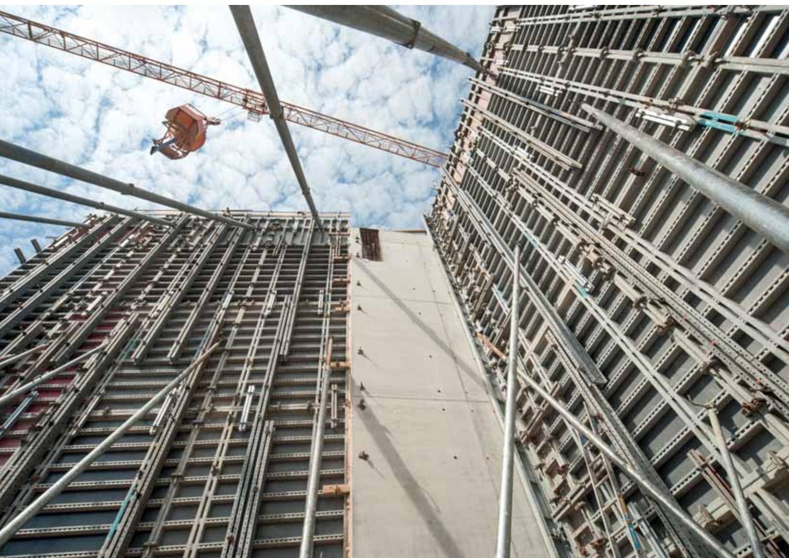
**Efficient concrete formwork for climbers** – One of Europe's largest climbing and bouldering centres is being constructed in Munich with NOEtop large area panels 2
