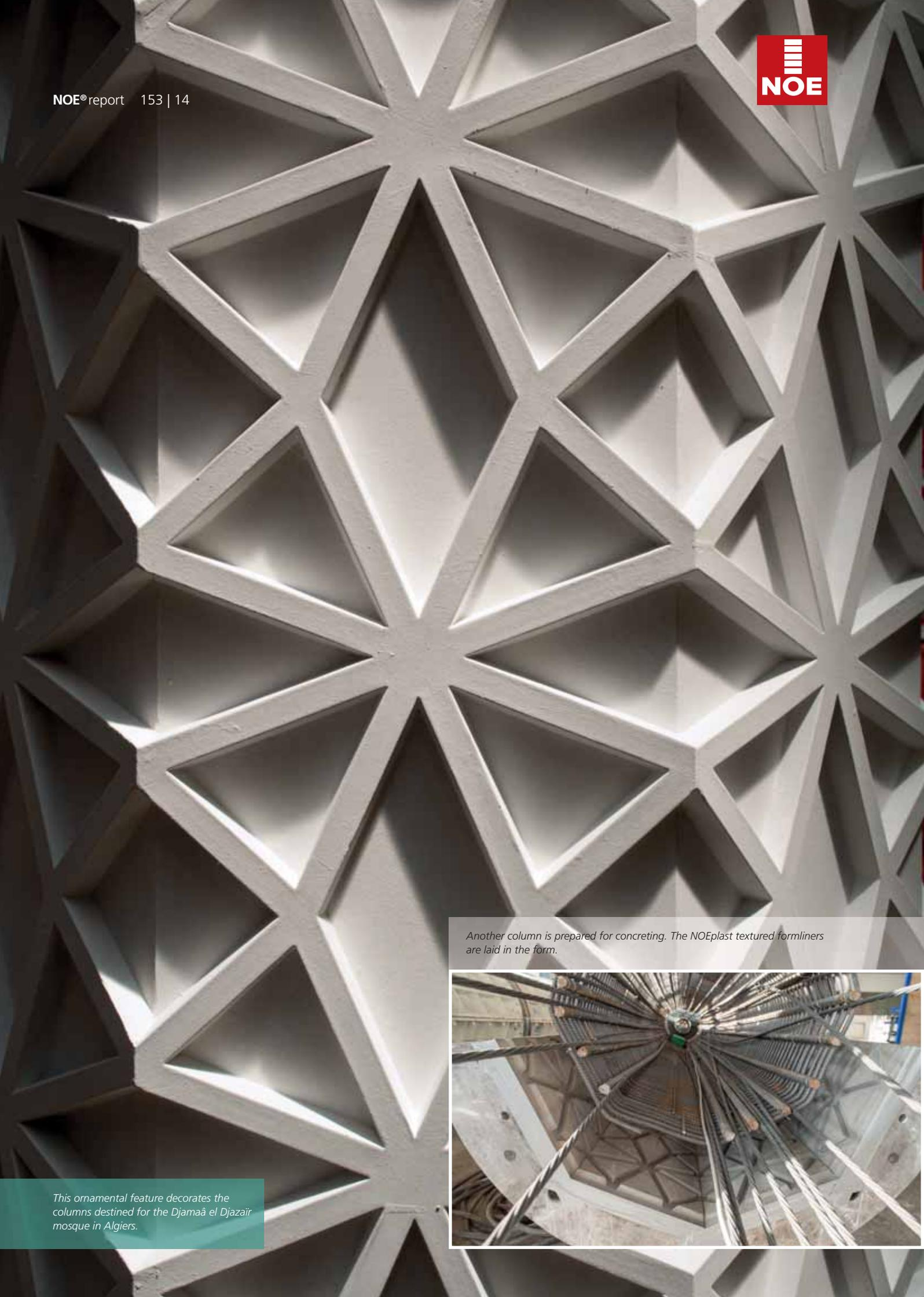
*Another column is prepared for concreting. The NOEplast textured formliners are laid in the form.*
