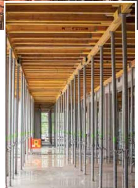
NOE H20 deck formwork rounds off the full service package for the Isoldenstrasse Housing Development project.
