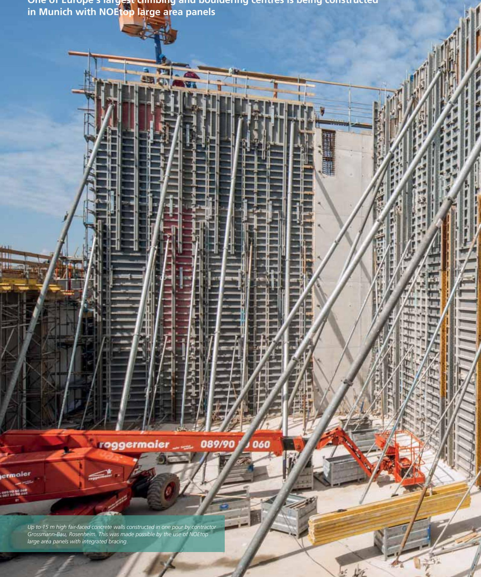
Up to 15 m high fair-faced concrete walls constructed in one pour by contractor Grossmann-Bau, Rosenheim. This was made possible by the use of NOEtop large area panels with integrated bracing.
