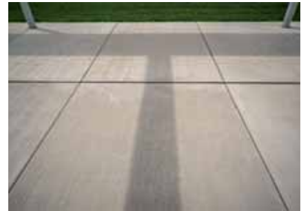
NOEplast Sydney: A delicately drawn brushed concrete texture on large precast concrete slabs.
