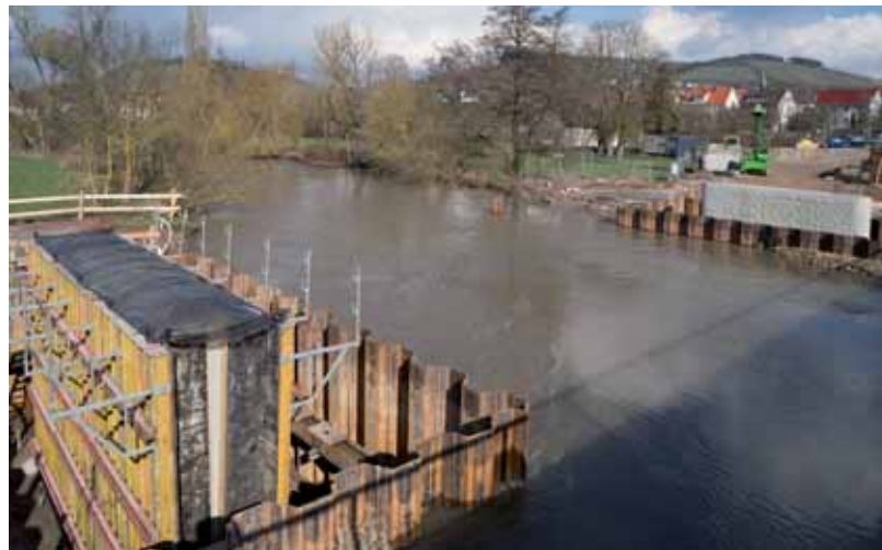
The concrete surfaces of the abutments were formed with NOEplast "Kufstein" masonry textured formliner.
