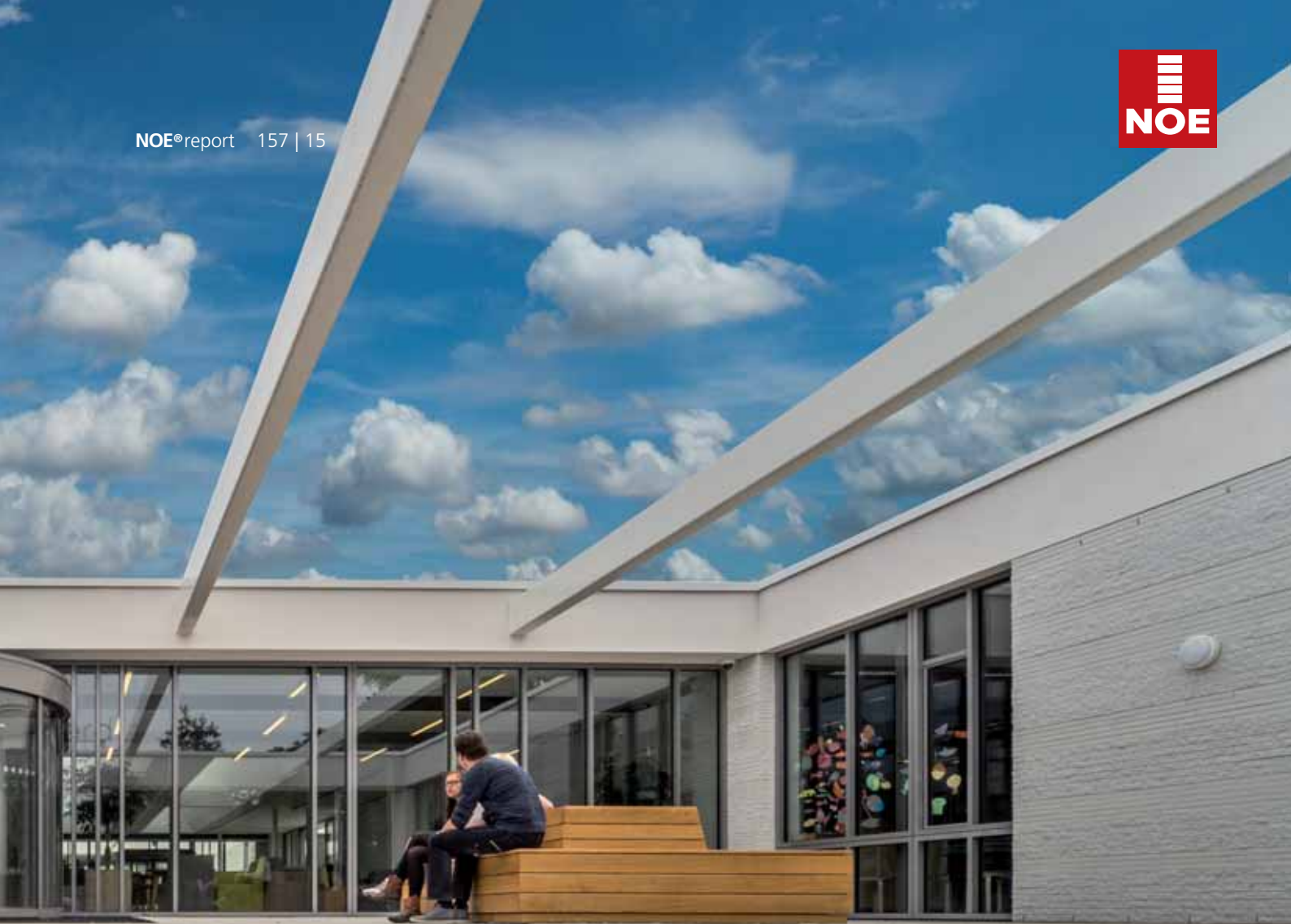
The traditional brushed finish is reproduced in the concrete using the NOEplast Sydney texture.
