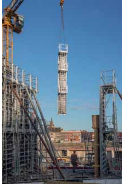
NOEtop S can be moved to the next position without the working platforms and access ladders having to be disassembled.
