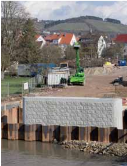
The concrete surfaces of the abutments and piers were formed with NOEplast "Kufstein" masonry textured formliner to look like natural stone cladding
