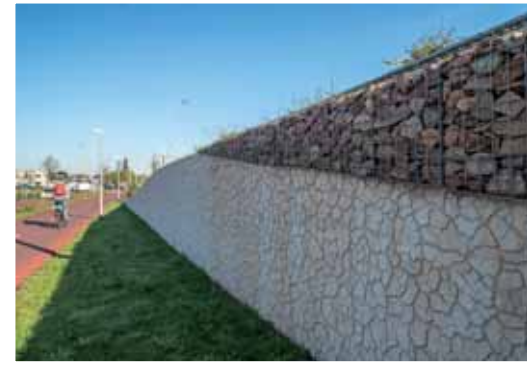
The features of a dried-out and cracked clay surface are reproduced on a retaining wall in Velsen, the Netherlands. Realised with the new NOEplast texture "Santpoort".
