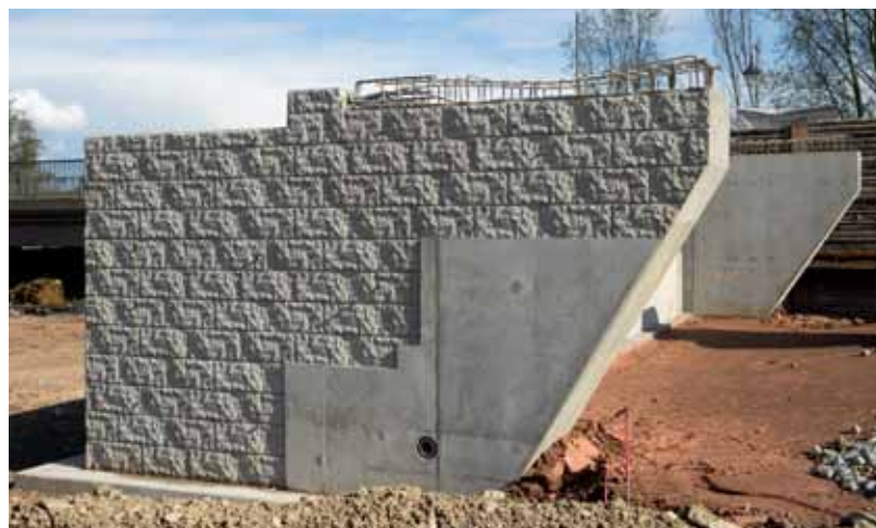
The concrete surfaces of the abutments were formed with NOEplast "Kufstein" masonry textured formliner.
