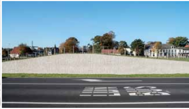
The face of this retaining wall in Velsen, the Netherlands, looks like a section through a low mound of earth, the exposed face of which has dried out. Realised with the new NOEplast texture "Santpoort".
