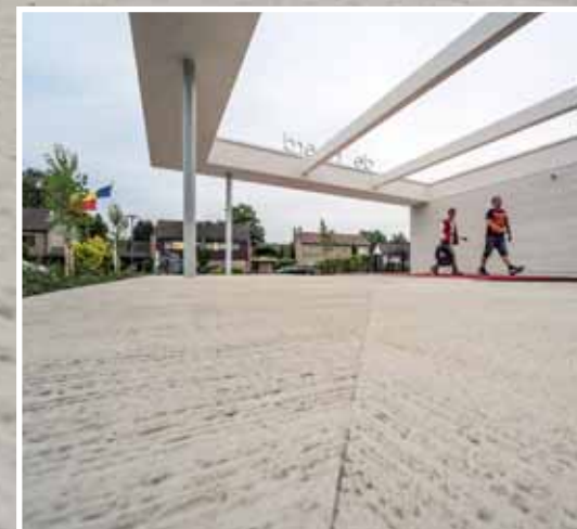
The traditional brushed finish is reproduced in the concrete using the NOEplast Sydney texture.
