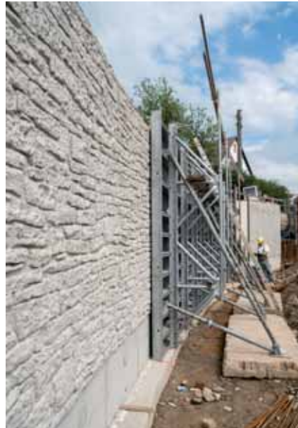
Tie-rod-free fair-faced concrete: with NOE Combi 70, the tie rods are positioned in the unseen plinth area and above the formwork.
