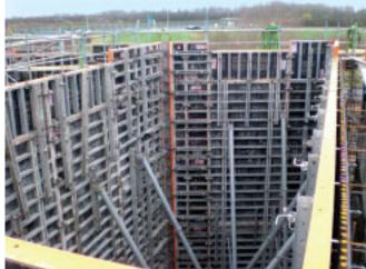
The panels are stabilized with NOE BKS push-pull props.
