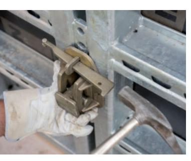
Fastening the swivel bearing that holds the tapering tie rod end on a NOEtop large area panel.
