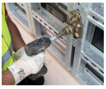
Use of the NOEtop EinsA with external tie rod bridge on a NOEtop standard panel.
