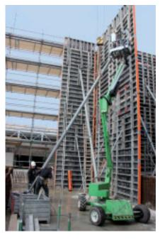
Imposing: 11.50 m form height, 0.60 m wall thickness and concreted in one pour in less than 36 hours.
