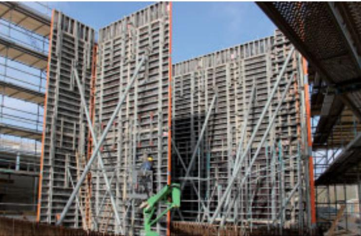
The panels are stabilized with NOE BKS push-pull props.
