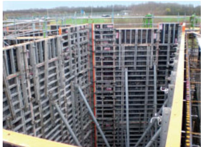
Impressive: only three NOEtop panels were required for over 30 m<sup>2</sup> form face.
