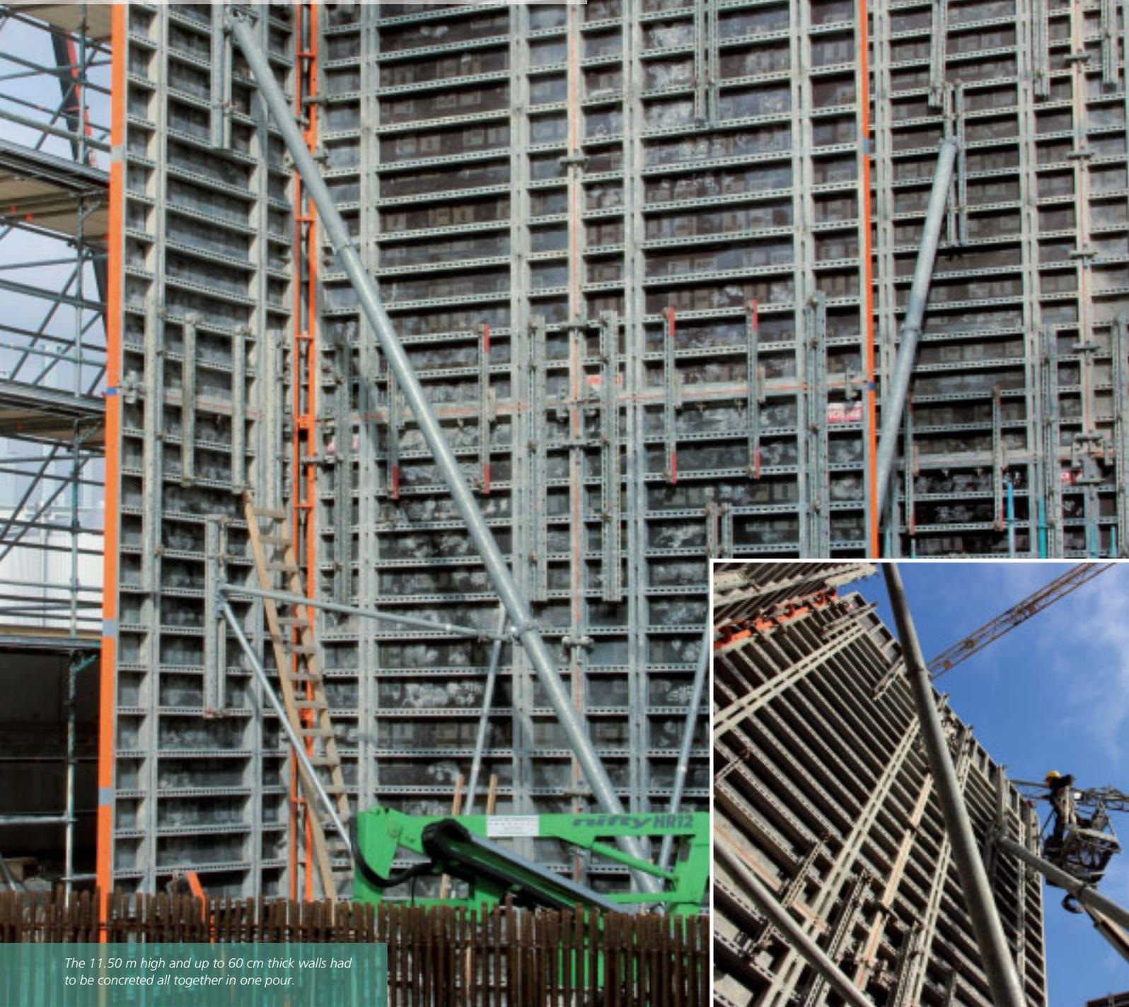
*The 11.50 m high and up to 60 cm thick walls had to be concreted all together in one pour.*
