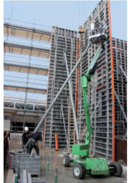
*Imposing: 11.50 m form height, 0.60 m wall thickness and concreted in one pour in less than 36 hours.*
