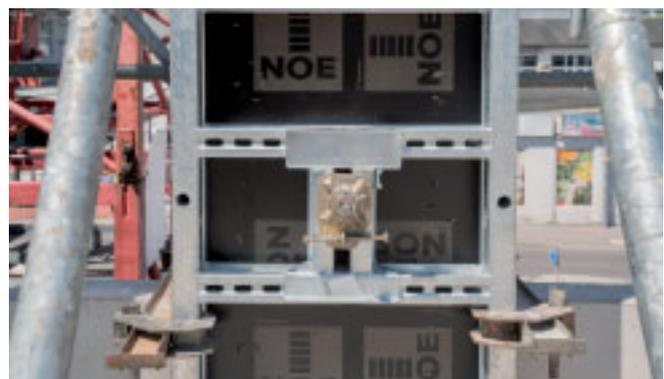
used tie rod holes to be sealed, nor is it required to erect scaffolding on the far side of the formwork to install the tie rods. Instead, the system has a simple clamping mechanism that can be preset using a 10 mm increment. This is how the required wall thickness is set. The process takes hardly any time at all. Cost-effective rubber seals ensure there are no leaks at the tie rods. The formwork can be operated completely from one side.
