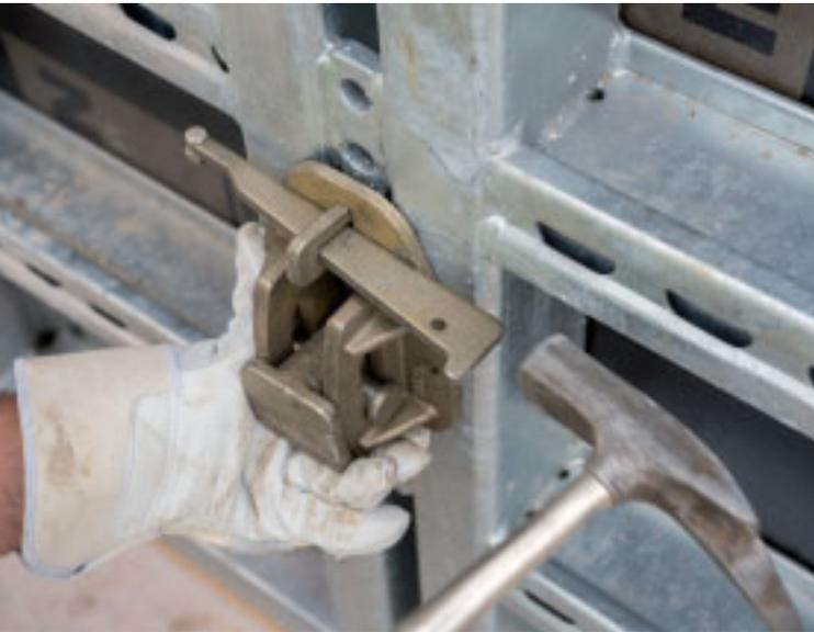
*Fastening the swivel bearing that holds the tapering tie rod end on a NOEtop large area panel.*
