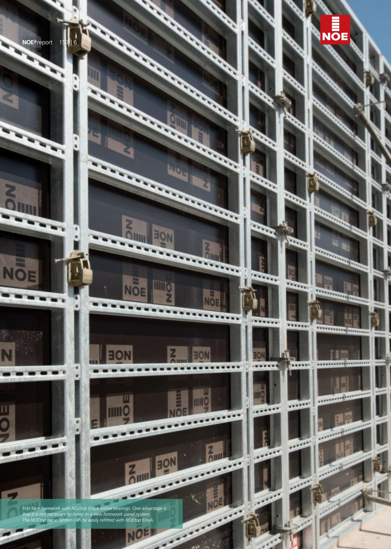
First face formwork with NOEtop EinsA swivel bearings. One advantage is that it is not necessary to invest in a new formwork panel system. The NOEtop panel system can be easily refitted with NOEtop EinsA.
