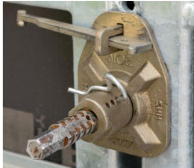
*The tapering tie rod can be preset in 10 mm increments using the NOEtop EinsA adjuster nut.*
