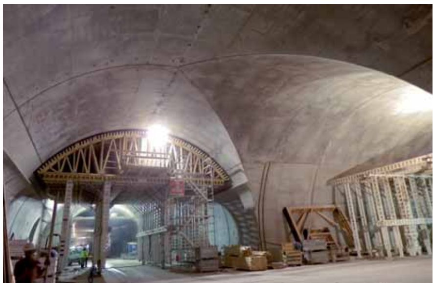
Finished ventilation gallery/tunnel tube intersection at emergency bay 2
