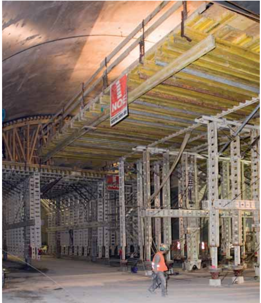
NOEtec formwork carriages for the emergency bay (left) and ventilation gallery (right)
