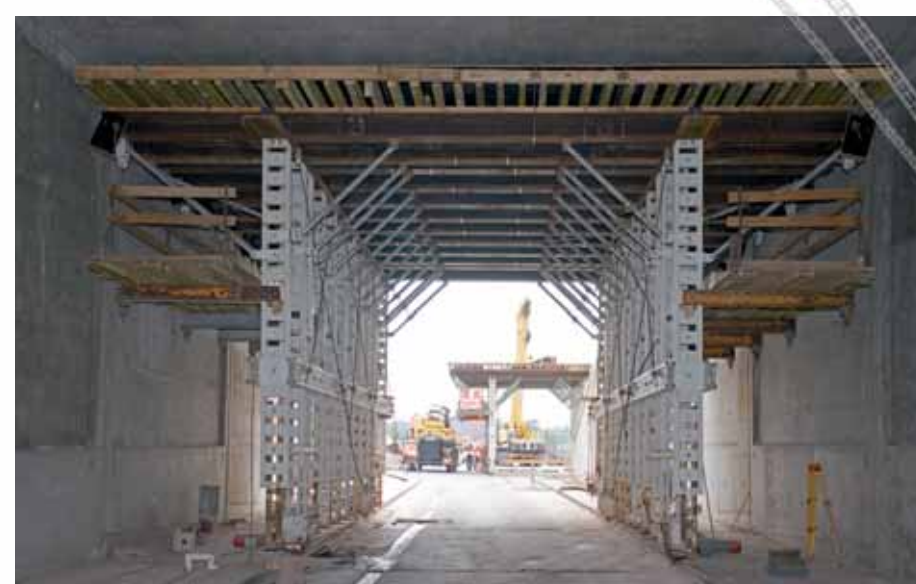
Cut-and-cover tunnel construction east: the formwork carriage in the background is being prepared for the move from the south to the north tube
