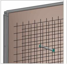
Push the plastic tube together with the support cone onto the tie rod recess tube of the first-face formwork, before or after fixing the reinforcement
