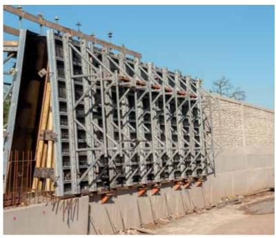
With the NOE Combi 70 system, the ties were placed in the plinth area and above the formwork. There were no ugly tie bar marks in the fair-faced concrete surfaces.
