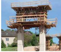
The 25 cm panel width of the NOEratio beam formwork proves itself of particular benefit on the slender cross section of the columns supporting the bridge over the Leutersbach valley.
