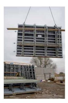
NOE Combi 70 – a formwork system primarily used in housing construction because the ties can be placed in the plinth area and above the formwork, which is perfect for places where smooth, wallpaper-ready concrete surfaces are required. At Cossebaude, this system was used to ensure the fair-faced concrete surfaces were free of tie bars.
