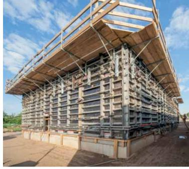
The panels had a max. size of 300 x 512.5 cm, so that 9.60 m long wall segments could be concreted using only 4 formwork panels.
