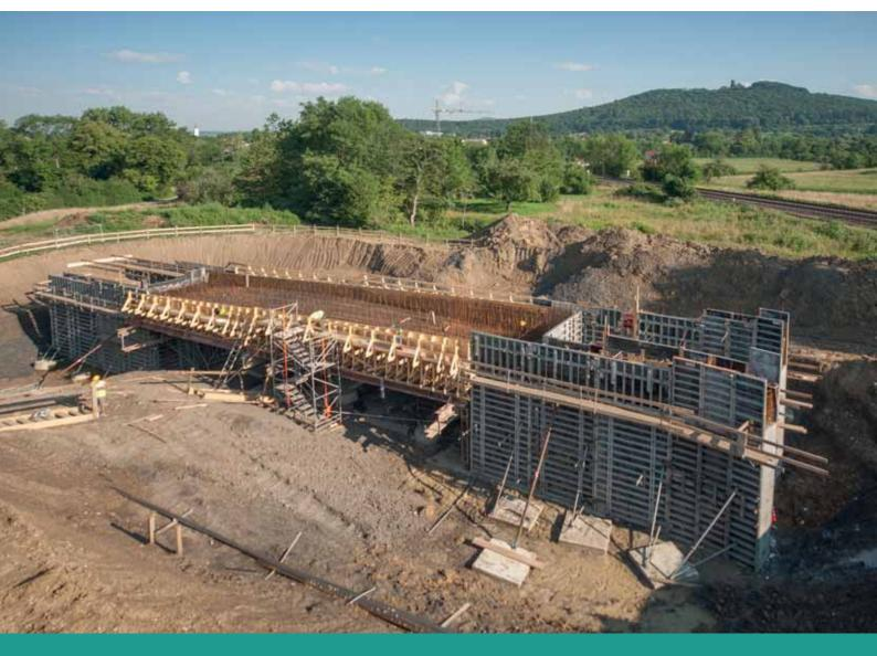
Concreted in one pour – NOEtop wall formwork allows a bridge to be concreted in one pour 2
