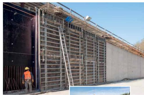
The tunnel portal walls were poured using NOEtop large panel formwork. The tie bar hole positions can be placed anywhere in the bracing.
