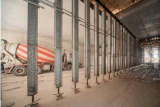
The temporary propping was performed by NOE LS 200 heavy-duty props.
