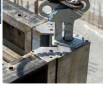
After release from the concrete surface, the internal formwork unit can be drawn slightly into itself by the
