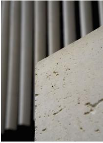
The ivory-coloured lisenes could be mistaken for natural travertine. Only a specialist would be able to tell the difference. The use of "Travertin" NOEplast textured formliners allowed any slight unevenness to be disquised.
