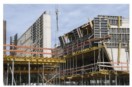
NOEtop frame formwork brings its big plus to bear in the extension of the Meilenwerk Böblingen: the well thought-out panel grid.
