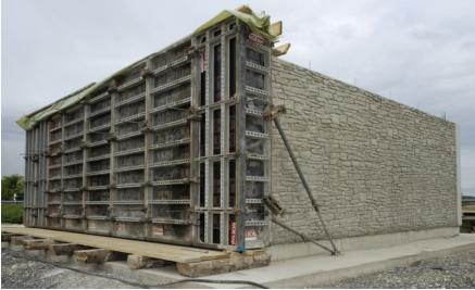
The NOE system components (formliners and formwork panels) complement each other excellently and thus ensure a perfect result.
