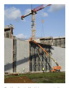
The side walls up to 13 m high were concreted in one operation.
