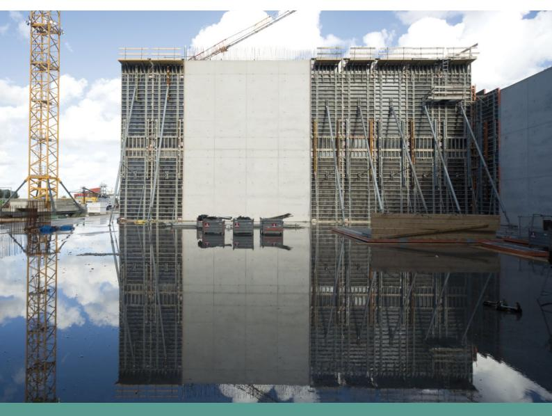
From nought to eighteen in two lifts 18 m high walls in only two concrete lifts 2 High horsepower in fine form Concrete, steel and glass – a new building for road horsepower enthusiasts 5
