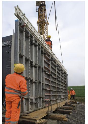
An ideal combination of NOEtop frame formwork and NOEplast textured formliners. The NOEplast Murus Romanus textured formliner was supplied attached to a supporting board by NOE.
