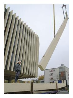
A logistical challenge: the transport and installation of the 13 m plus long lisenes on Ingolstadt Nord station in possibly windy conditions.
