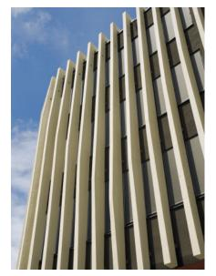
The surface of the lisenes looks like the natural stone travertine. This appearance was created by placing NOEplast textured formliners in the precast concrete unit forms. Architect Zurmöhle remarked: "... the concrete surface always looked simply perfect."
